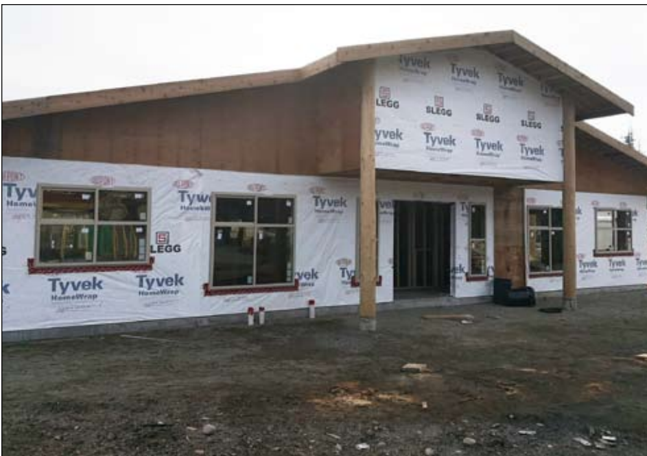
The new Daycare building is getting very close to completion
