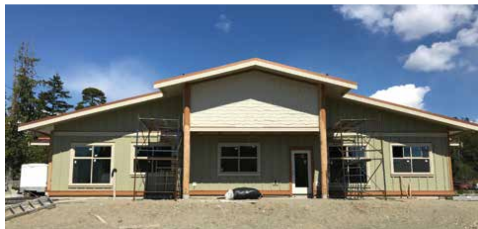
New Daycare building almost ready for occupancy
