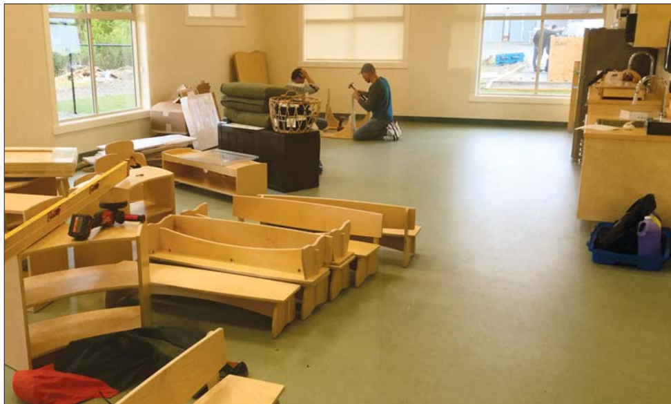
Workers prepare benches for inside the new Daycare building.
