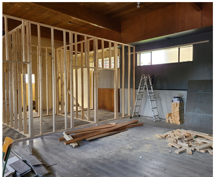
These photos, during renovation, show the wall taken down to the existing office space as shown above. New framing as been put to create additional office space and peeking through the framing, renovations to the bathroom are also underway.
