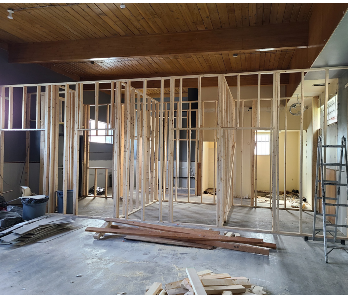
These photos, during renovation, show the wall taken down to the existing office space as shown above. New framing as been put to create additional office space and peeking through the framing, renovations to the bathroom are also underway.
