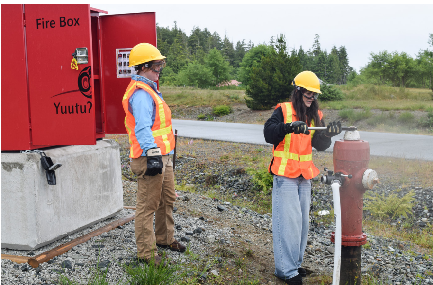
Rose Aday and Katie Burden, Fire Box trained volunteers, turn off the hydrant using tools from the Fire Box.
